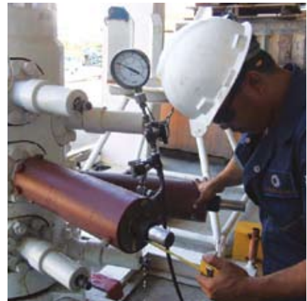
Wellhead Maintenance in progress
