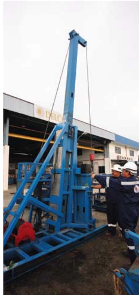
Erecting the wireline mast
