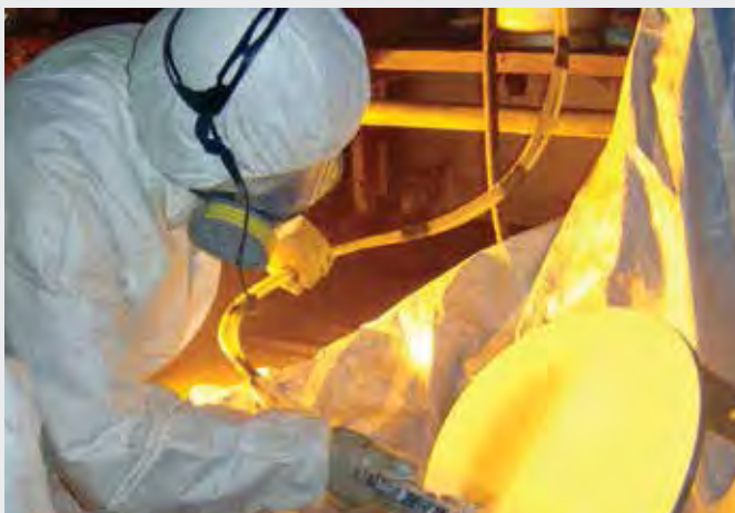
Internal lining coating
