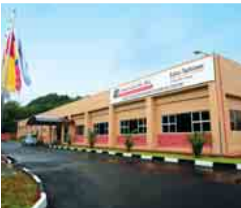
Turboservices Facility: Tuanku Jaafar Industrial Park, Negeri Sembilan.
