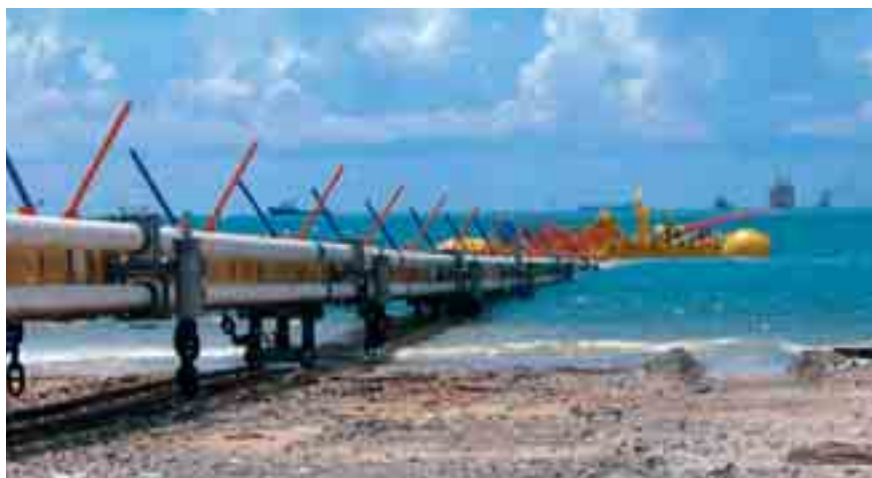
Launching of FTL pipe bundle from the Bintulu fabrication site.
